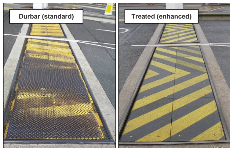
Figure 2: Blockers fitted with standard Durbar plates and with plates coated with a skid resistant surface treatment.
